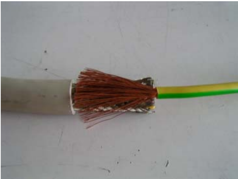
Fig. 3.2: Fan out the wires of the PE conductor and lay them on the shield
