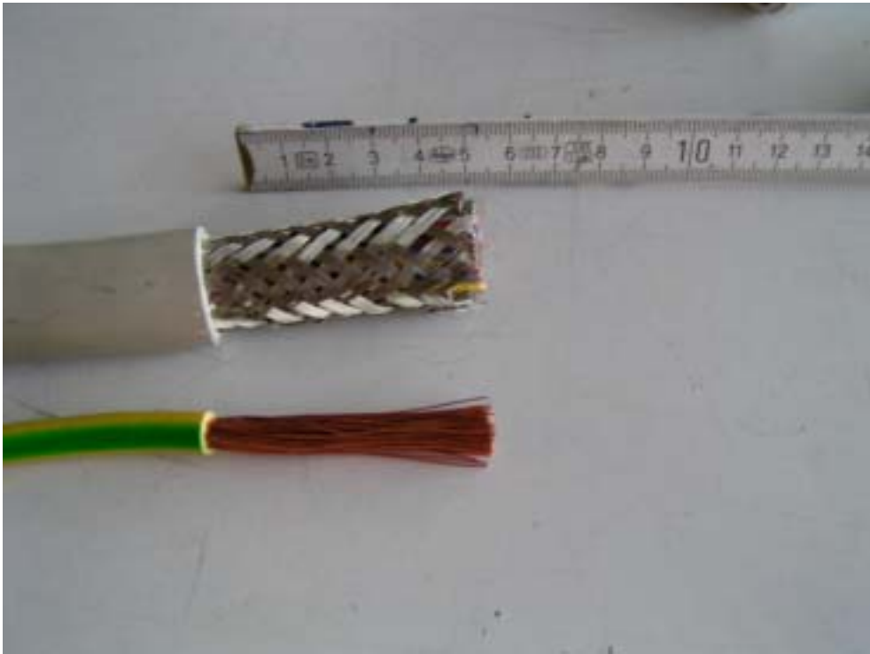
Fig. 3.1: Remove the insulation of e.g. JE-LIYCY 32x2x0.5 cable for contact force spring SA KRF 22 V2A and PE conductor 1x16 mm \leq (stranded) by approx. 5 cm in length.
