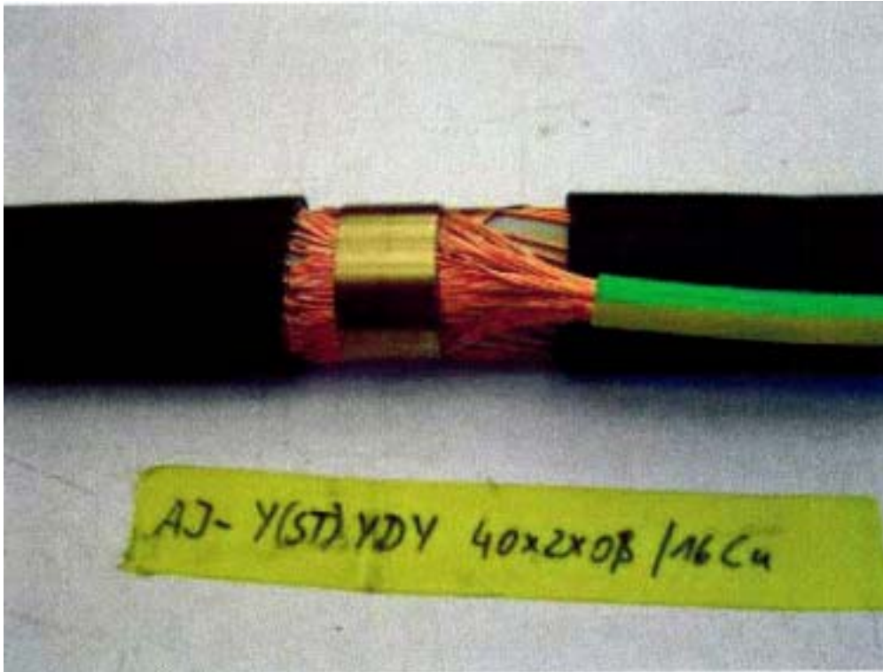
Fig. 2.3: Wrap the contact force spring SA KRF 29 V2A around both cables.
