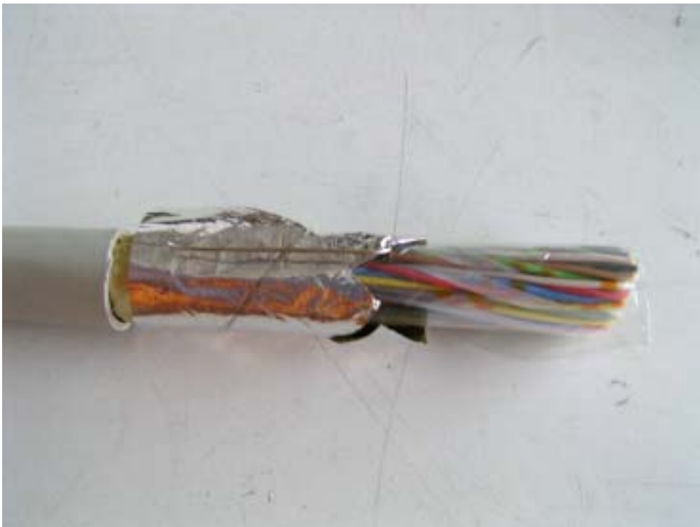
Fig. 4.2: Open the foil and sheath wire and turn over approx. half of the uninsulated area
