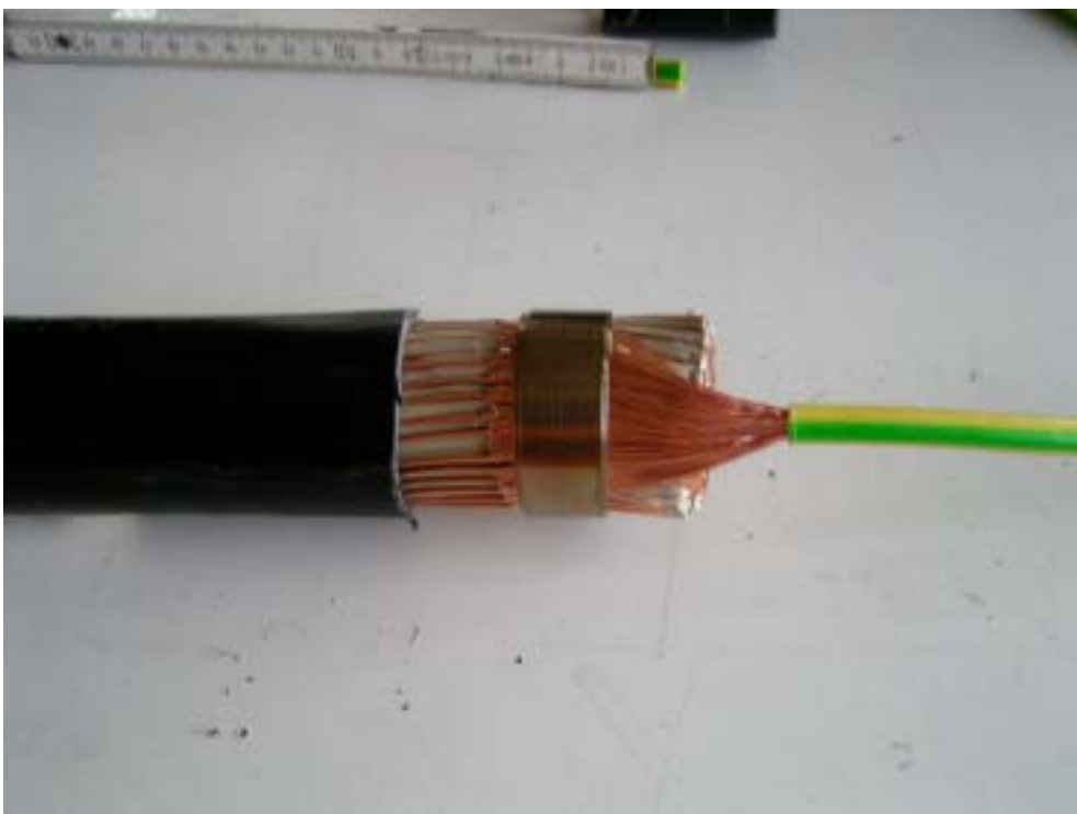
Fig. 1.4: Contact force spring completely mounted
