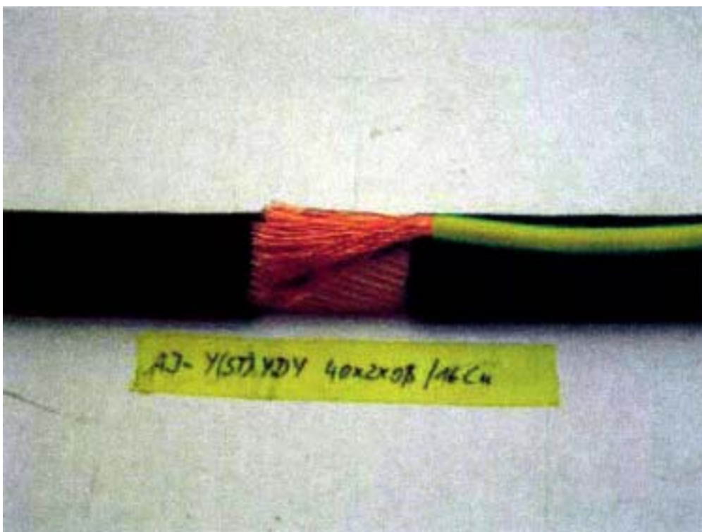
Fig. 2.2: Fan out the wires of the PE conductor and lay them on the shielding
