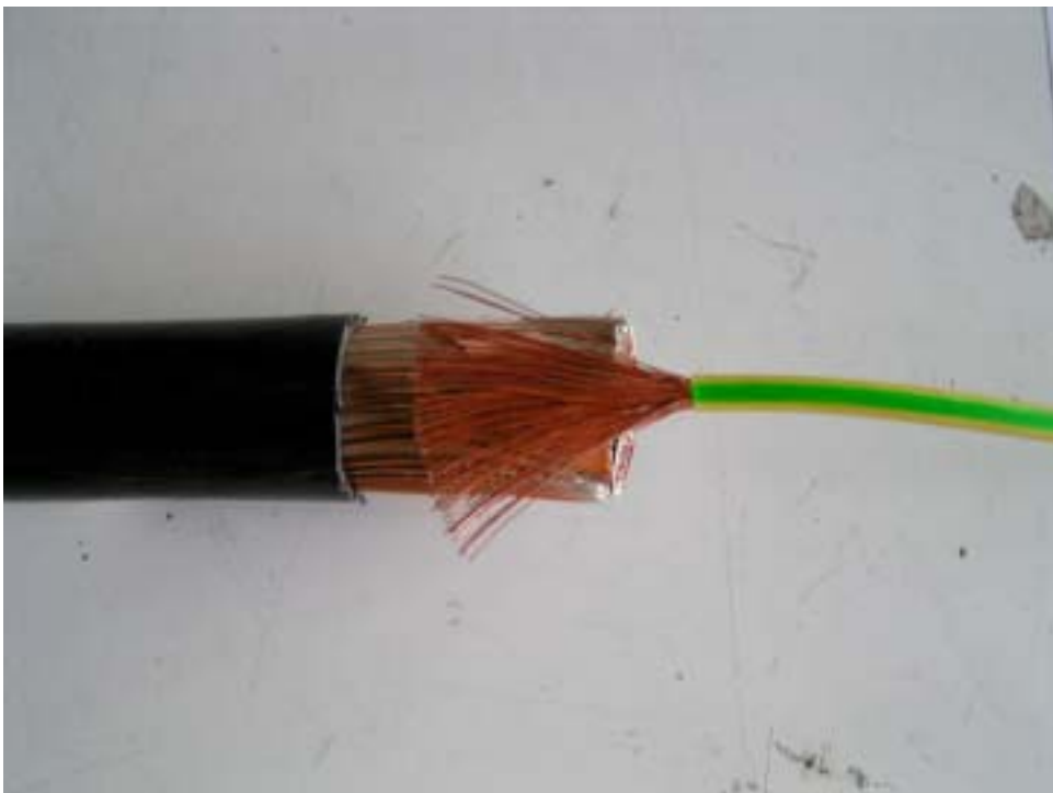
Fig. 1.2: Fan out the wires of the PE conductor and lay them on the shield.
