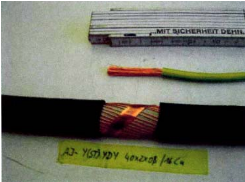
Fig. 2.1: Remove the insulation of e.g. AJ-Y(ST)YDY 40x2x0.8/16 Cu cable for contact force spring SA KRF 29 V2A and PE conductor 1x16 mm \leq (stranded) by approx. 5 cm in length.
