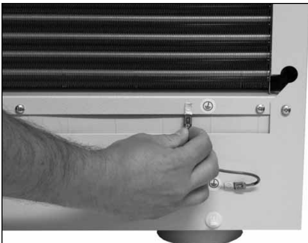
Fig. 22: Disconnect the earthing cable
