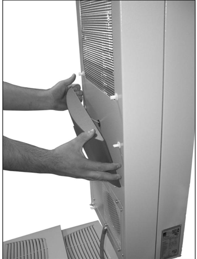
Fig. 37: Remove the infill panel
