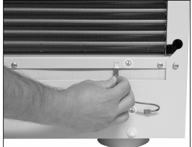
Fig. 25: Disconnect the earthing cable
