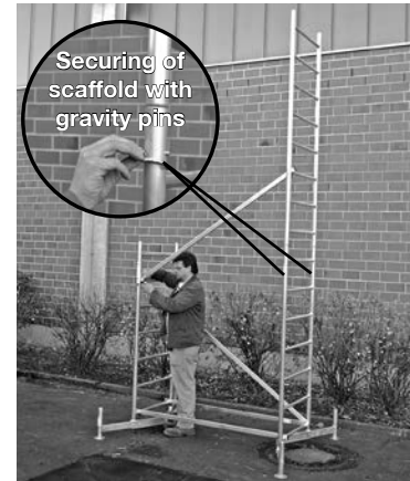
Basic scaffold with first extension
