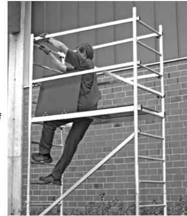
Basic scaffold with first extension
