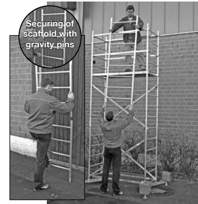
Basic scaffold with first and second extension
