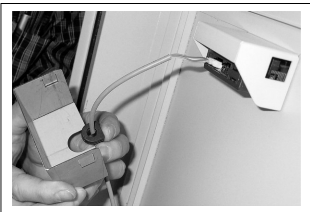
Fig. 14: Insert the cable sleeve
