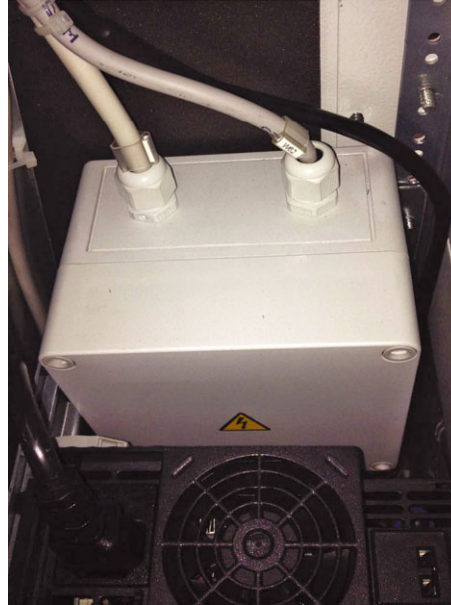
Fig. 50: Additional box for the thermal protection of the electrical heaters
