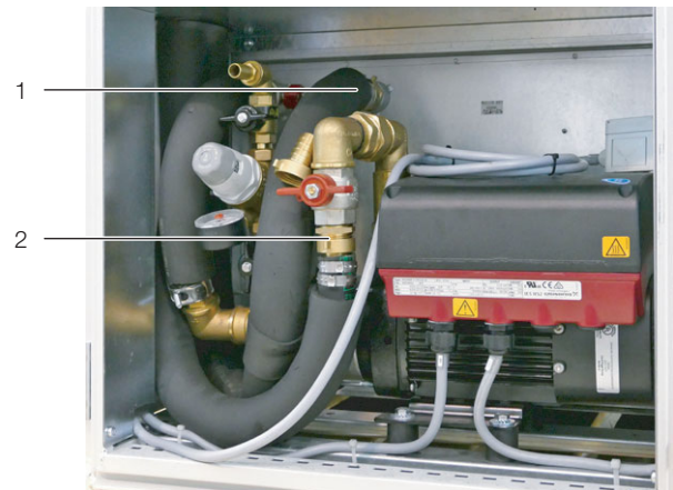
Fig. 20: Connection points at the bottom of the unit
