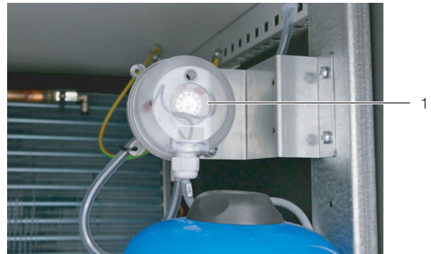
Fig. 60: Adjustment screw at the differential pressure sensor
